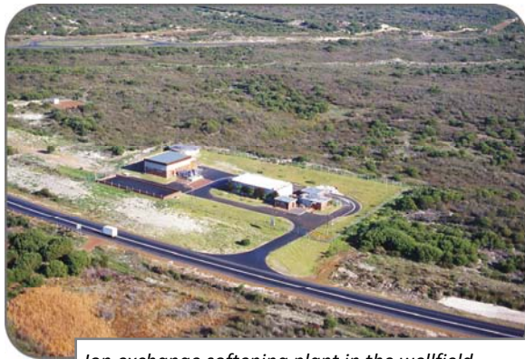
Ion exchange softening plant in the wellfield.
