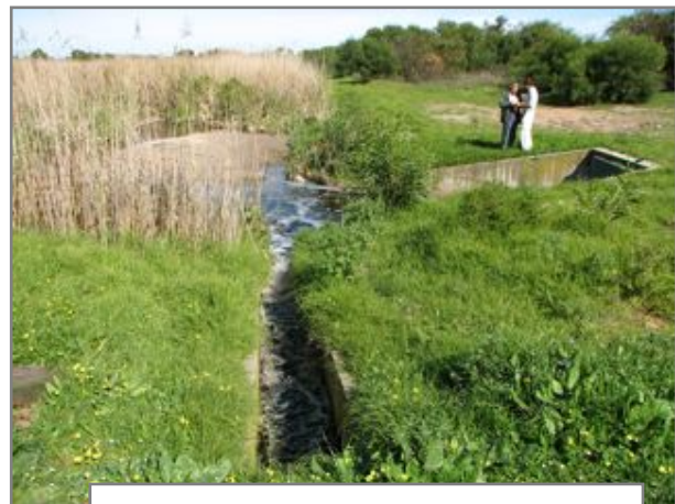
Basin 6: Inlet from treated domestic effluent (centre) and large diameter inlet from storm water collection system (right).
