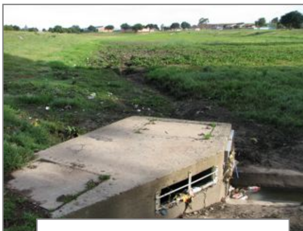
Basin 3: Storm water outlet.
