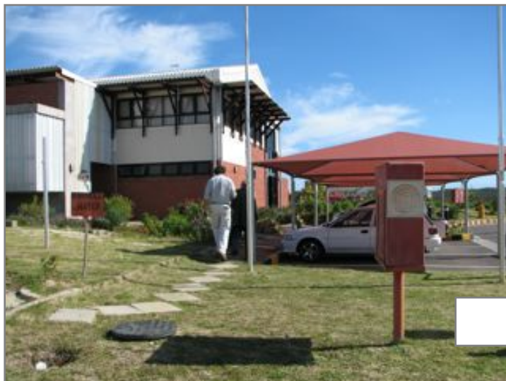
Softening Plant Office Block.
