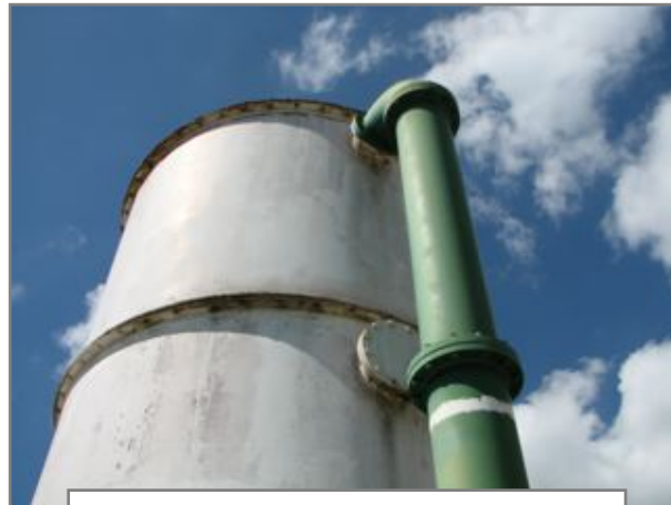
De-gassing chamber.
