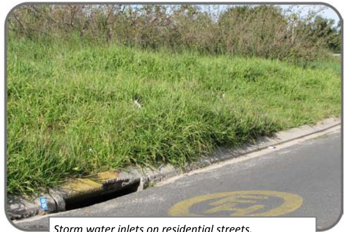
Storm water inlets on residential streets.
