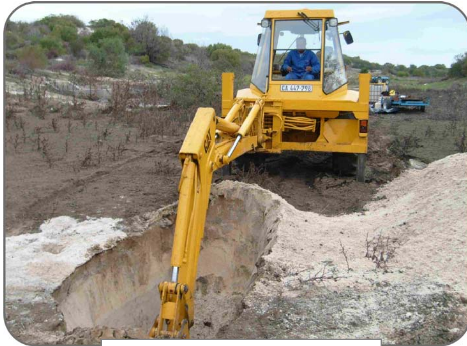
Basin 12 sand sampling - thin silt layer.
