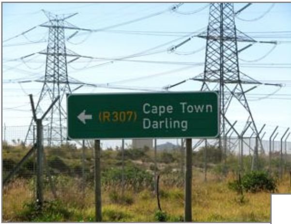
En route to Softening Plant.
