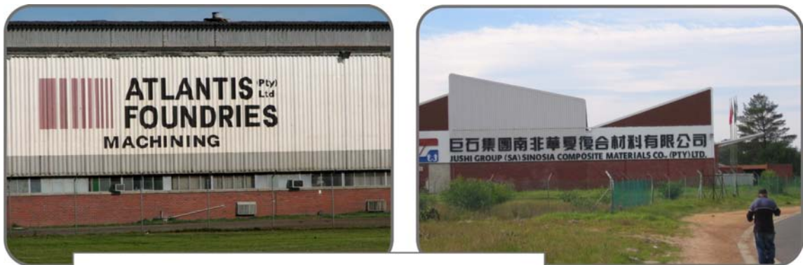
Industrial area of Atlantis.
