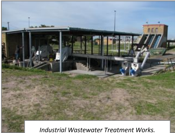
Industrial Wastewater Treatment Works.
