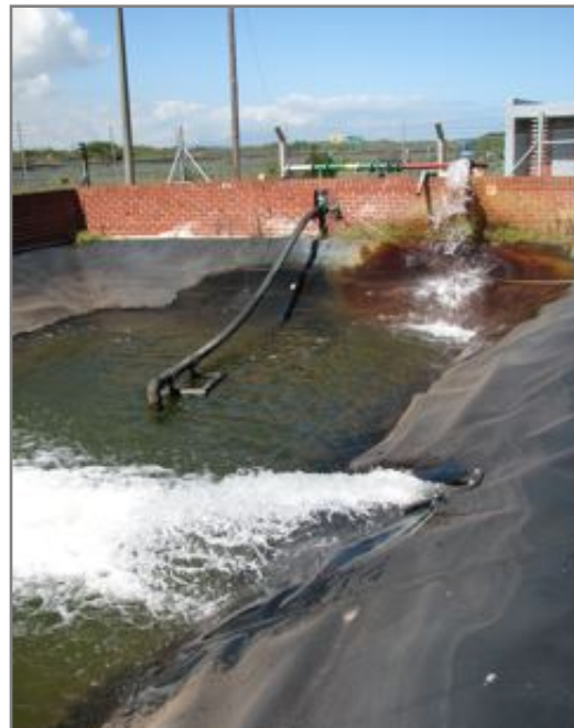
Waste acid pond: backwash brine from regeneration process (right); dilution water from borehole (back right); disposal pipeline suction (black pipe).
