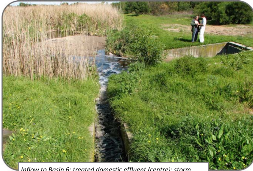
Inflow to Basin 6: treated domestic effluent (centre); storm water (right); with sediment deposits showing on left.
