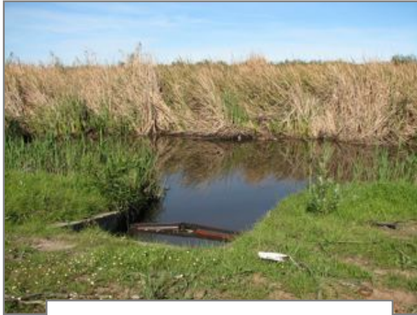
Basin 9: Industrial storm water detention.
