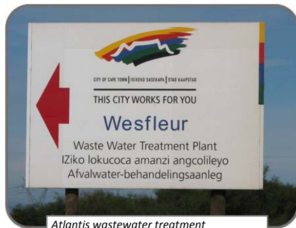
Atlantis wastewater treatment works.
