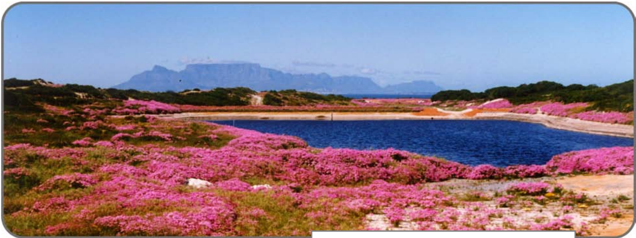
Coastal infiltration basin.
